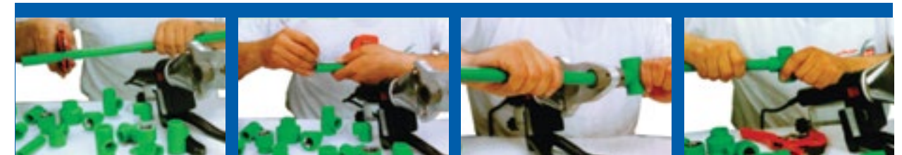
Welding Depth, Heating, Welding and Cooling Time
